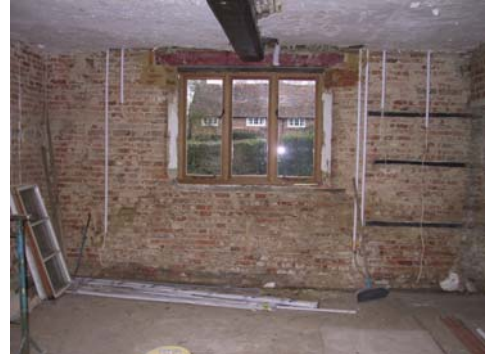
Services chased into existing wall
