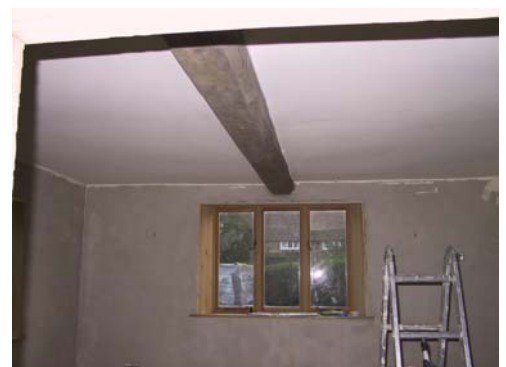
Baunit-Bayosan lime finish plaster onto the boards.
