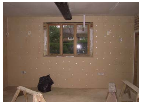
Pavatex Woodfibre boards applied over Baunit-Bayosan lime levelling coat of plaster.
